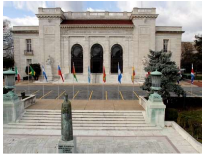
OAS Building, Washington D.C., USA
